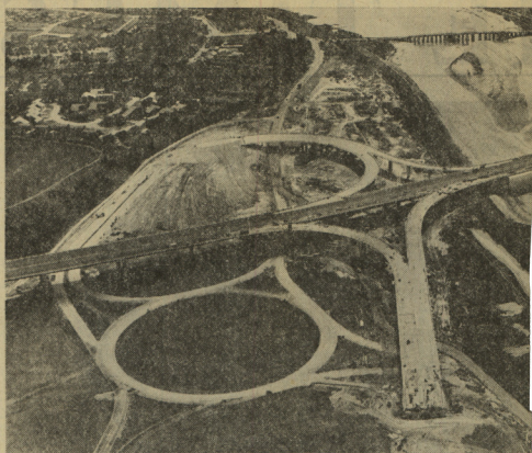
The Adur bridge and Shoreham by-pass which is part of the A 27 Folkestone to Honiton trunk road is in the background.
